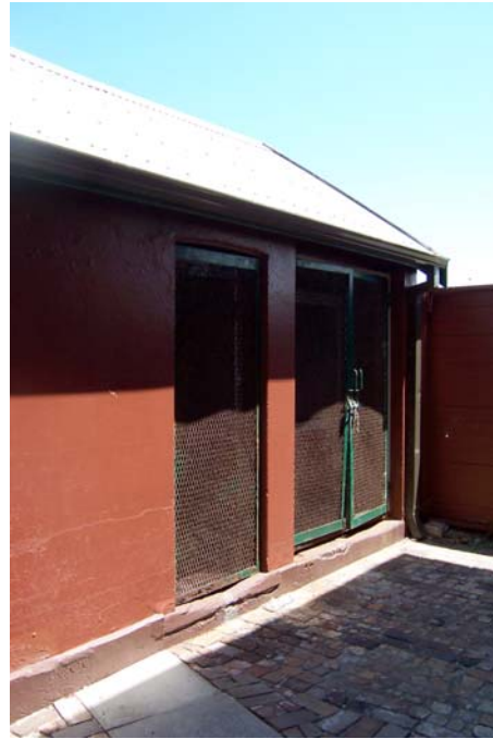
Fig. 4.1 View of Store Room from courtyard.
