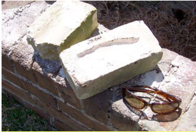
Fig. 3.7 Battery Room bricks with bullet-shaped frog.
