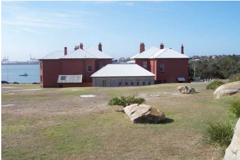
Fig. 2.6 View of Cable Station building complex from the southeast.
