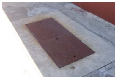
Fig. 5.8 (right) One of the two in-ground pits in the Courtyard.
