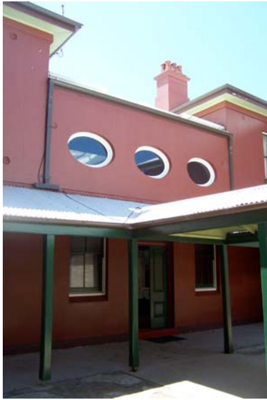
Fig. 5.2 (left) Location of the gutter spreader from the Instrument Room roof.
