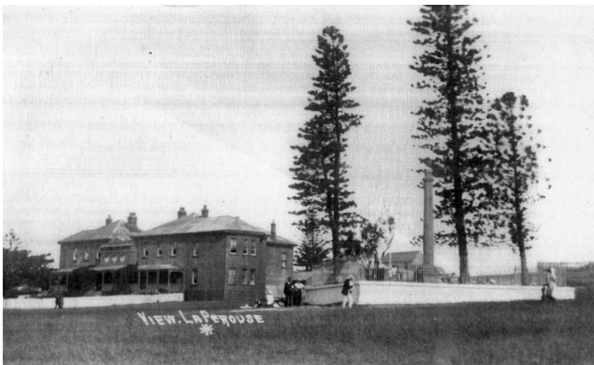
Fig. 6.13 View of the La Perouse Monument with Cable Station building in the distance. Tentatively dated 1906-1917 (Tuck: 174).
