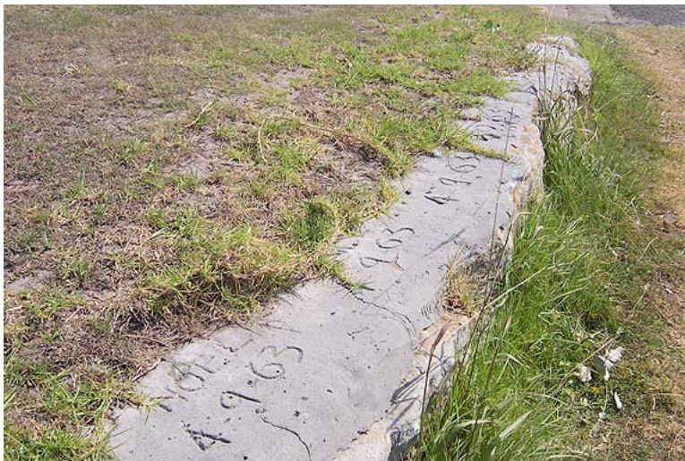
Fig. 8.9 Row of workers' initials at loop road retaining wall to the southwest of the Cable Station building. The Loop road circumscribing the Historic monument Reserve was completed in 1963.
