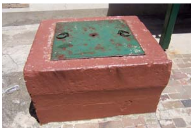
Fig. 5.7 (left) Painted concrete well with steel sheet cover.
