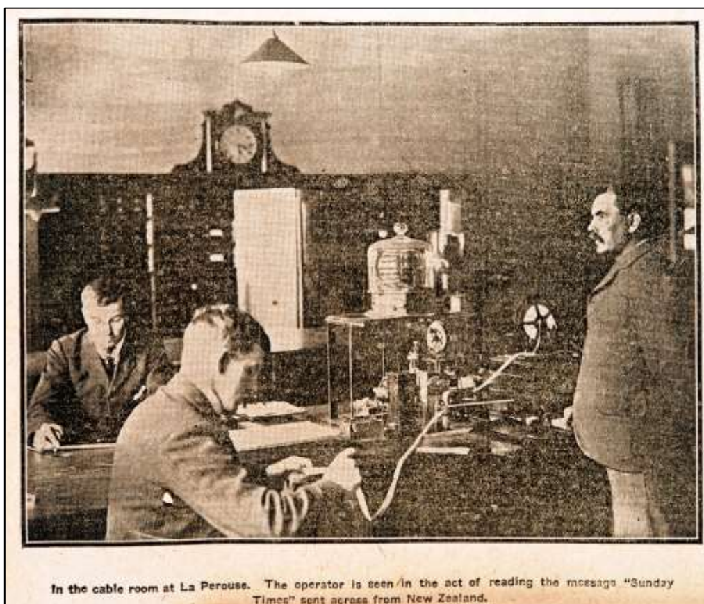
Figure 40 Yarra Bay House cable room, 1908
