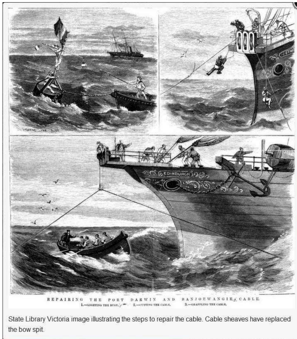
Figure 6 Repairing the Java to Port Darwin cable
