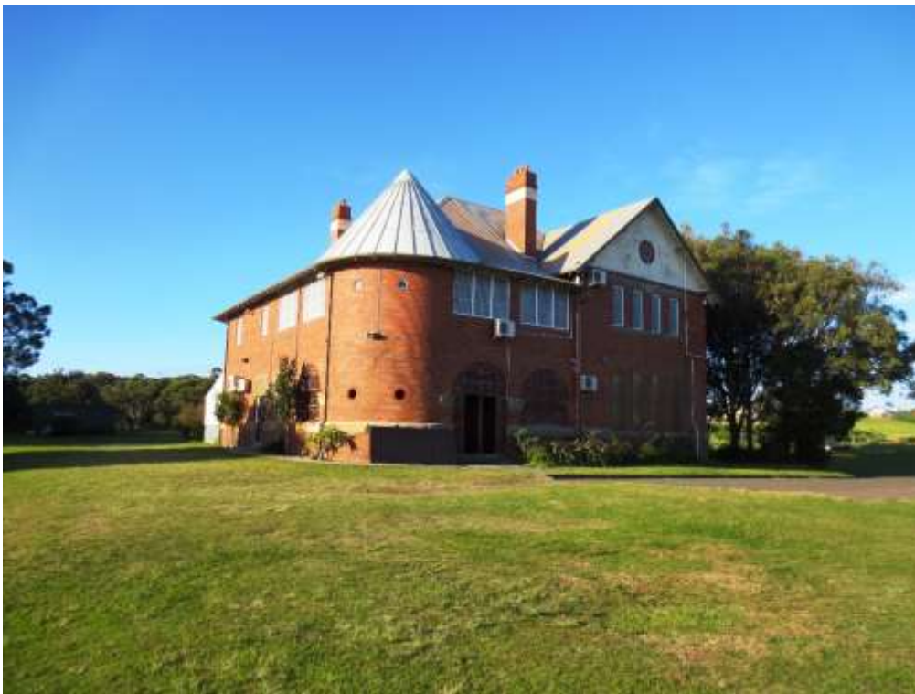
Figure 39 Yarra Bay House
