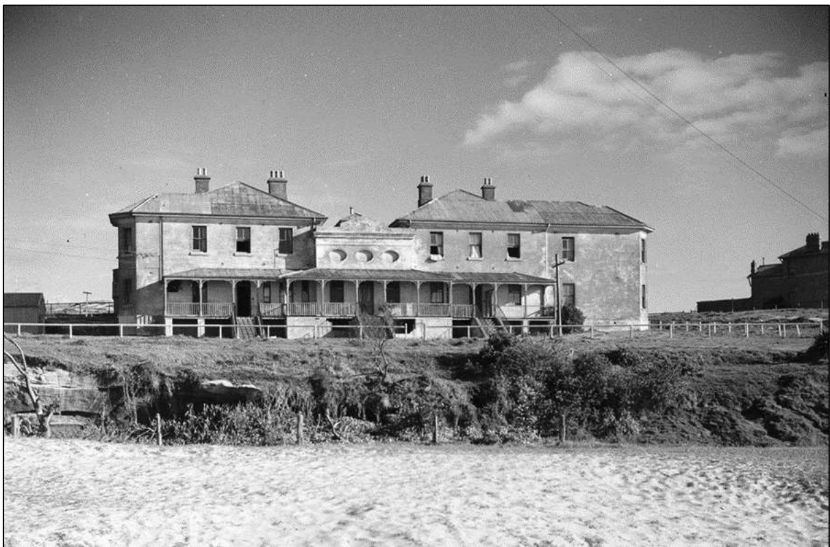
Figure 26 Cable Station, c1953 (Max Dupain)
