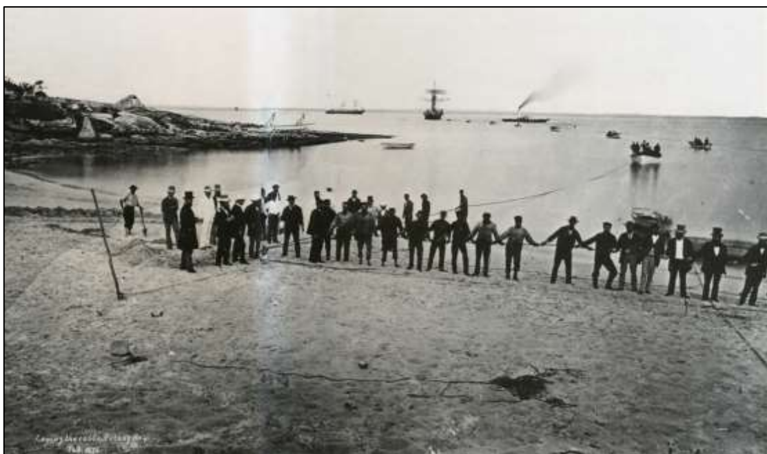
Figure 13 Laying the cable at La Perouse, 5 February 1876
