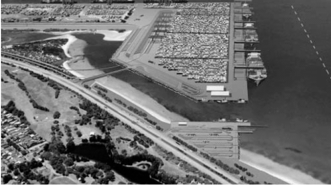
2011 view of new Port terminal, Boat and Tug Ramp, and Penrhyn
